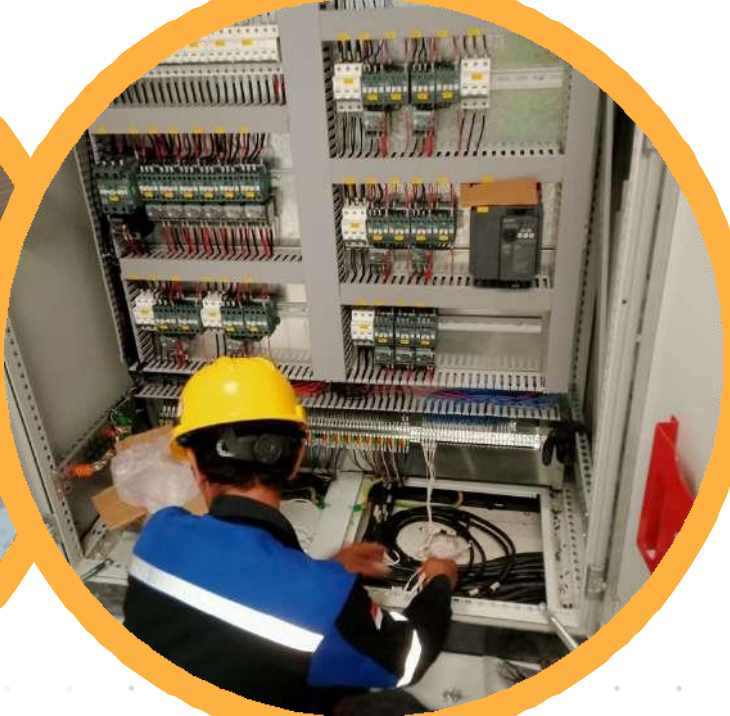
ELECTRICAL WORKS-WIRING CONTROL PANEL MDP SDP AND TERMINATION
